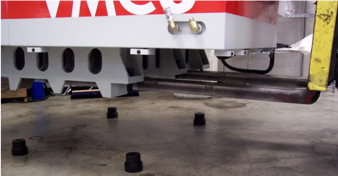
Figure 3 – Lifting the VMC
