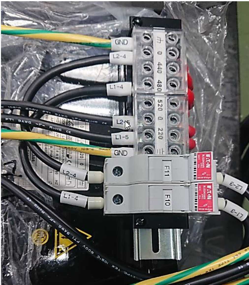
Figure 2.8.1 - Transformer Used on 480 Volt Machines
