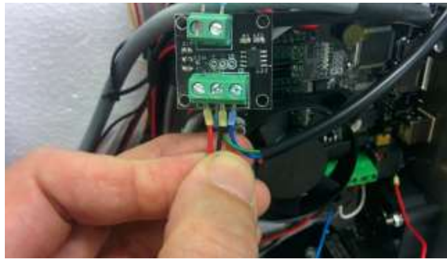
Figure 4.31.7 Connecting Leads from Auxiliary Power Supply
