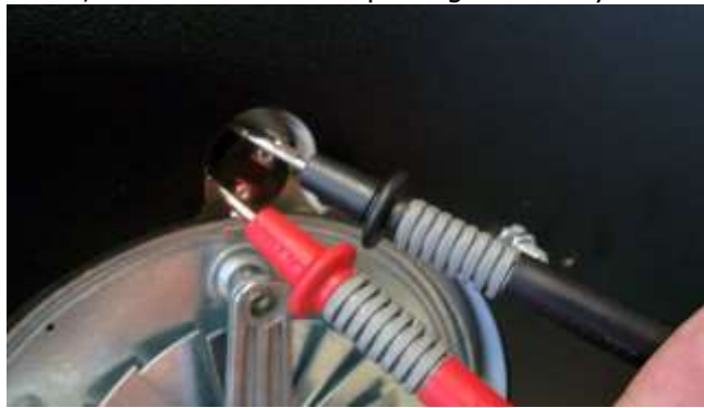
Figure 4.2.9 Checking Safety Thermostat Current
