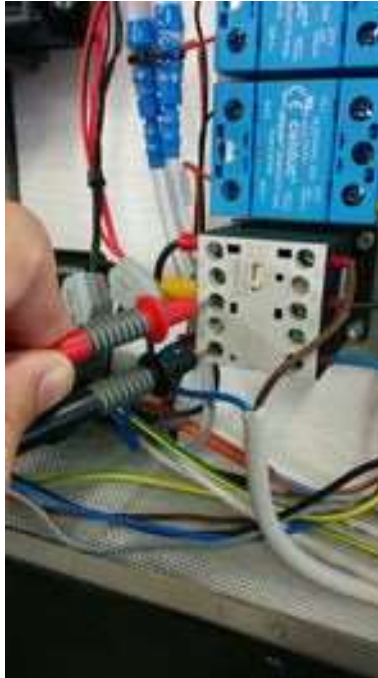
Figure 4.44.1 Testing AC Voltage on Contactor Entry
