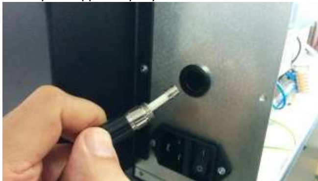
Figure 4.2.5 Checking Fuse on Main Switch
