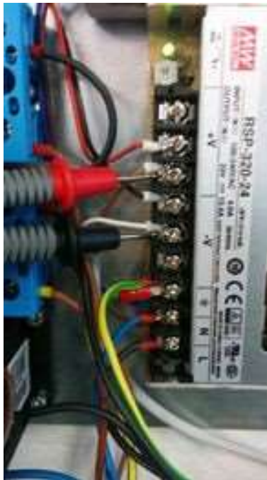
Figure 4.44.3 Testing 24V DC output on PSU Terminals
