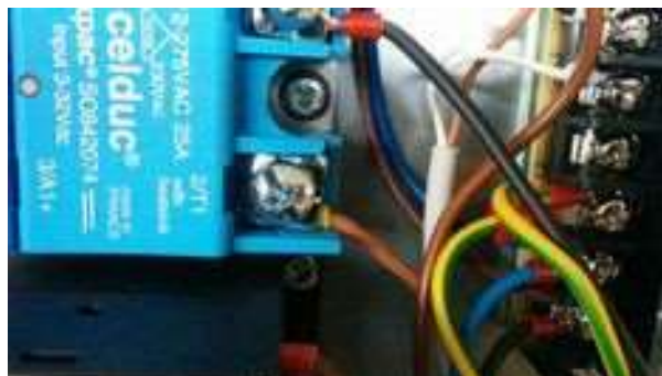
Figure 4.15.6 Incorrect SSR Cabling Connection
