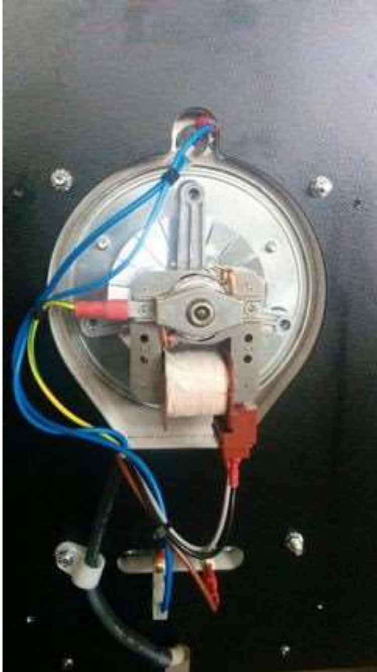
Figure 4.15.2 Fan Connections (Cover Removed)
