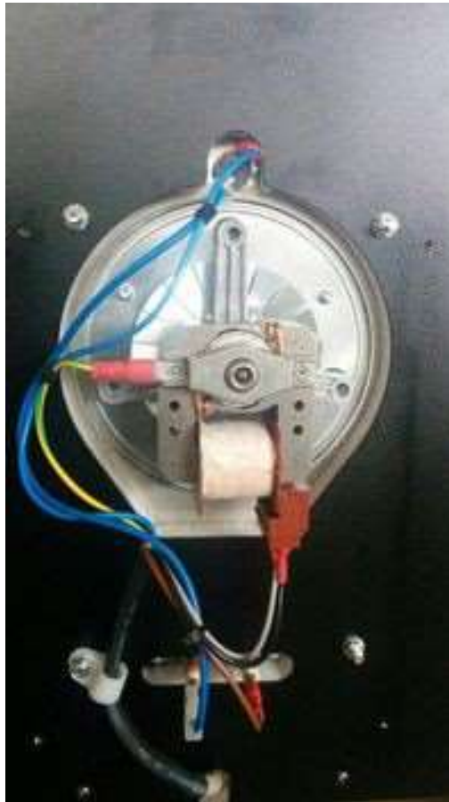
Figure 4.2.7 HC Fan Cover Removed
