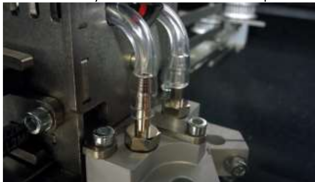
Figure 4.7.5 Coolant Piping after Replacement
