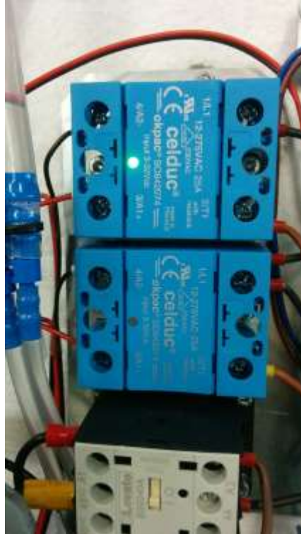
Figure 4.15.3 LED on Heated Chamber SSR
