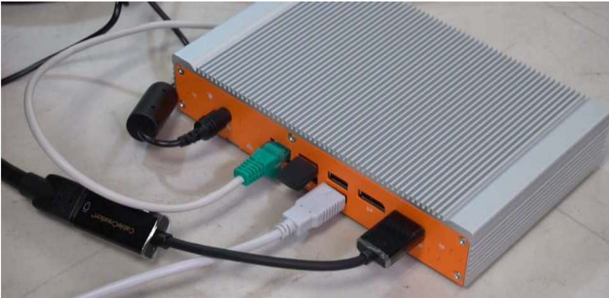
Figure 5.16.1 Print Server & Cables
