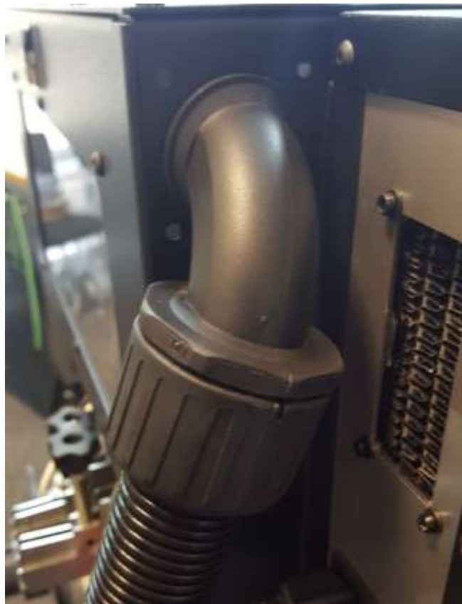
Figure 5.3.7 HEPA Filter 90° Elbow Adapter Installed
