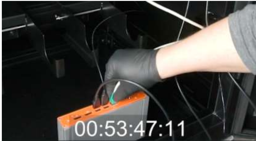
Figure 5.16.6 Cable Connections to Print Server within MMS
