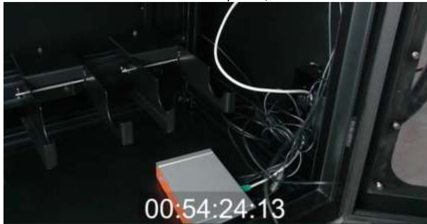
Figure 5.16.7 Printer Server and Cables within MMS
