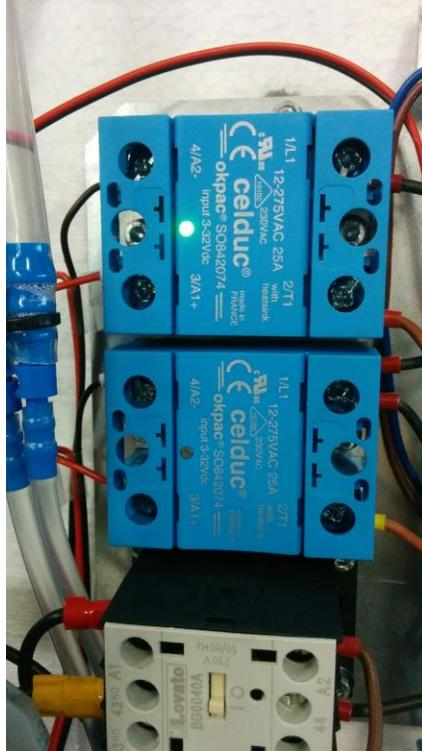
**LED on Heated Chamber SSR**
