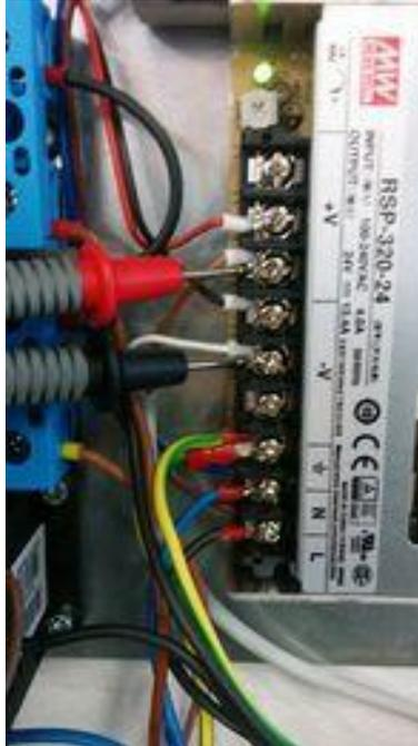
**Figure 6.24.3 Testing 24V DC output on PSU Terminals**
